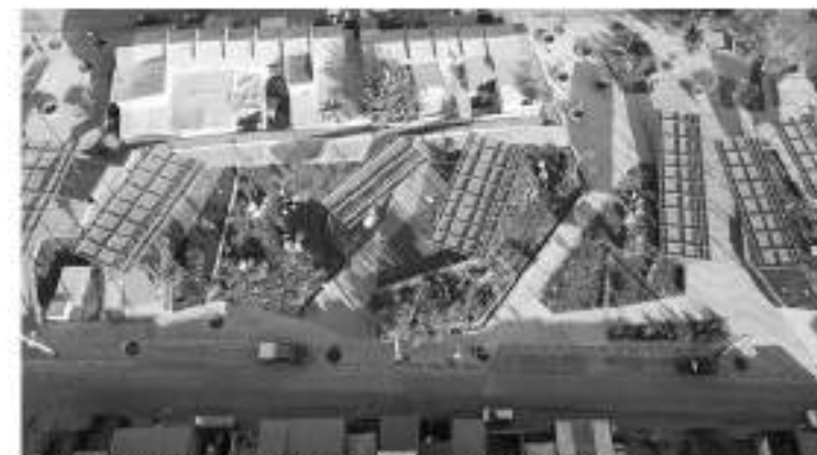
2.23 aerial image of the park (Archdaily, 2021)
