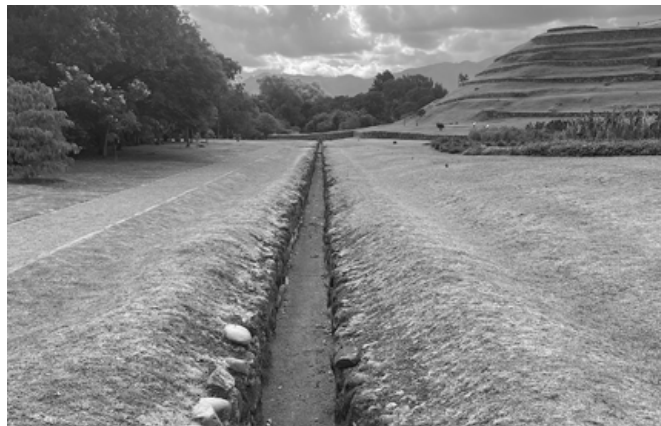
graphic 10: The prime relic: a canal built by the Incas to transport water from the río Tomebamba to the city.
