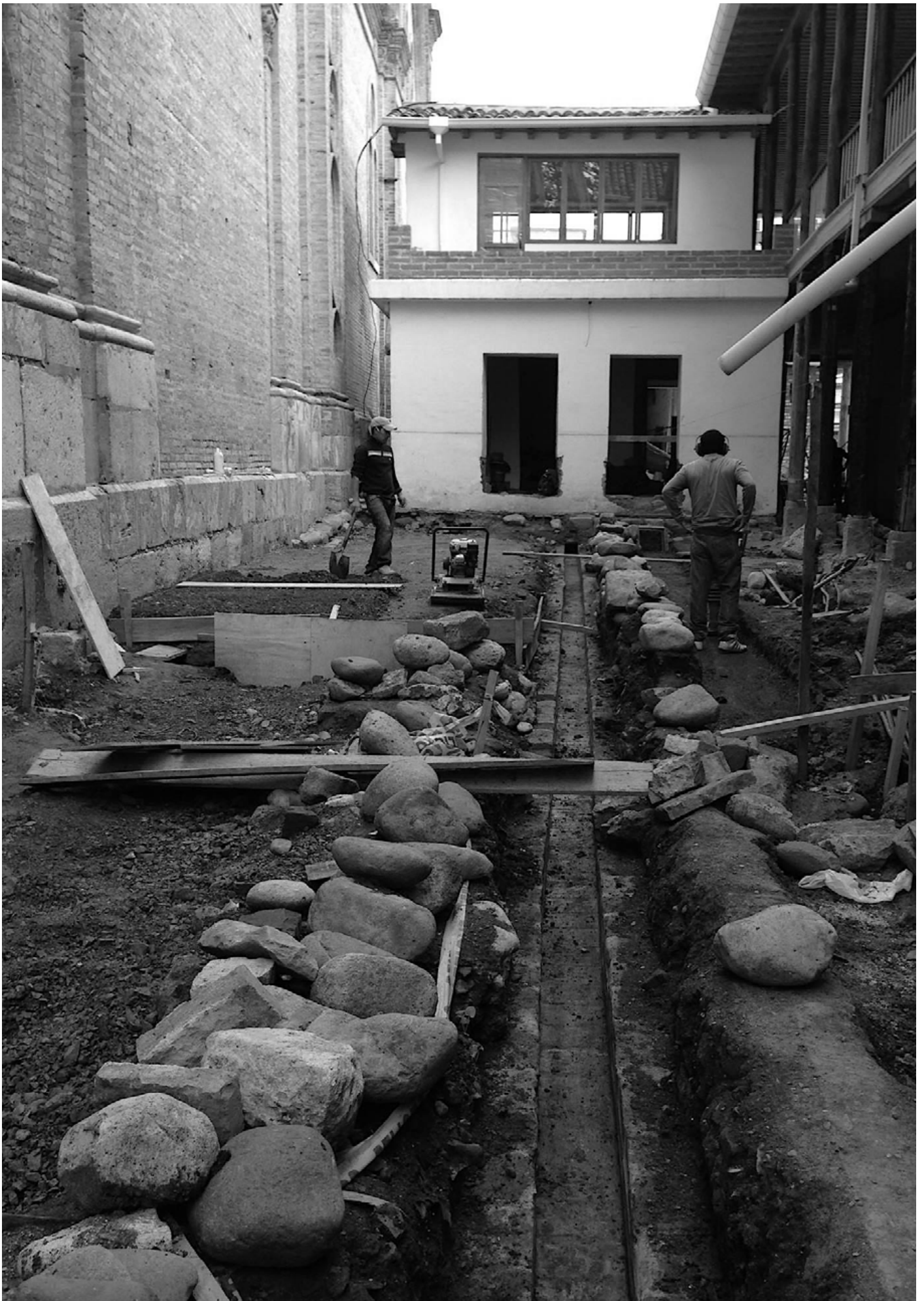
graphic 17: Construction site where an old canal is visible.
