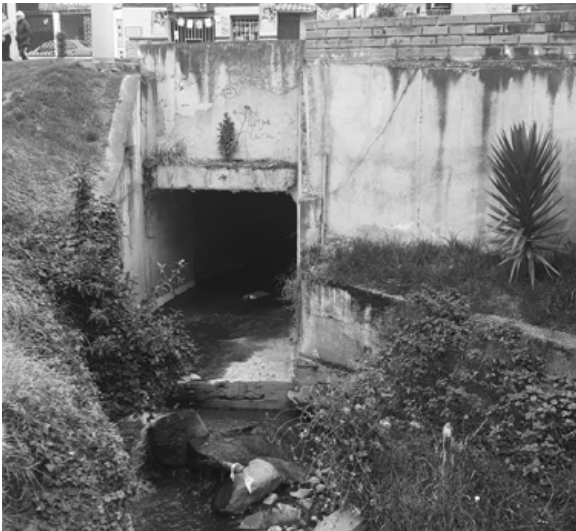
1. Quebrada Sacay Channelized
