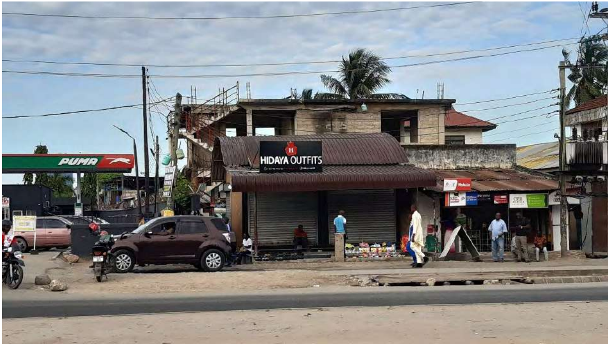
Fig. 2.5 - A vertical extension of commercial building at Mlalakuwa. [source: Fieldwork, 2022]
