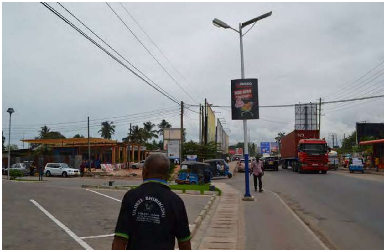
Fig.2. 8 – Makongo Juu Road: Mlalakuwa on the left, Mlimani City Mall on the right looking toward the crossover with Sam Nujoma road. [source: KU Leuven Summer Internship – Global Minds – VLIR-OUS project, (2022)]
